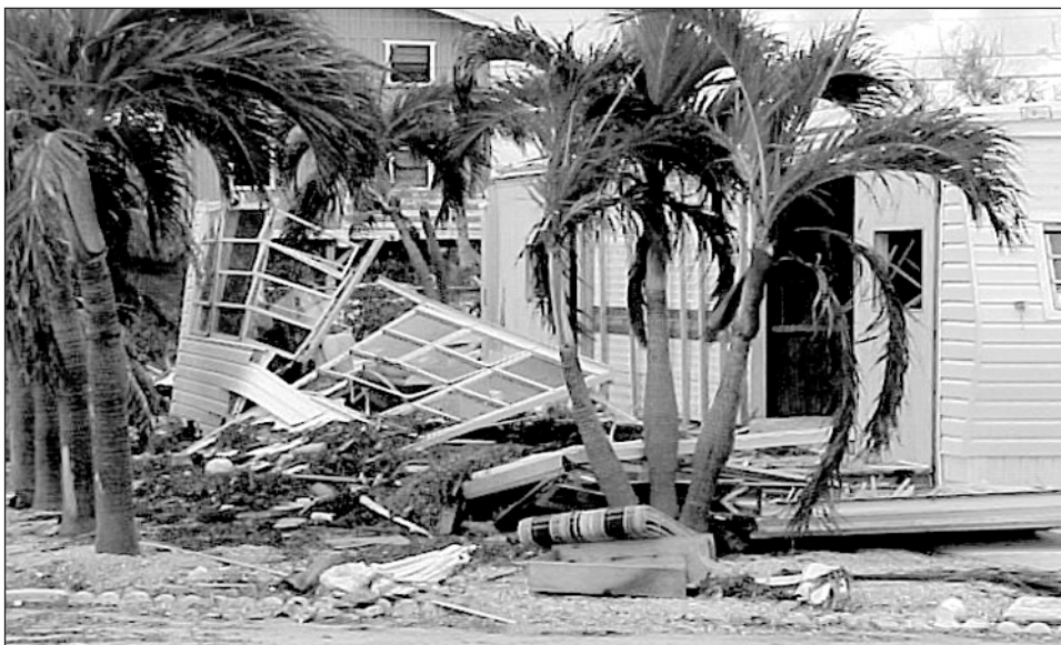
Figure 1-3. The addition to this manufactured home was destroyed, causing considerable damage to the rest of the home.
