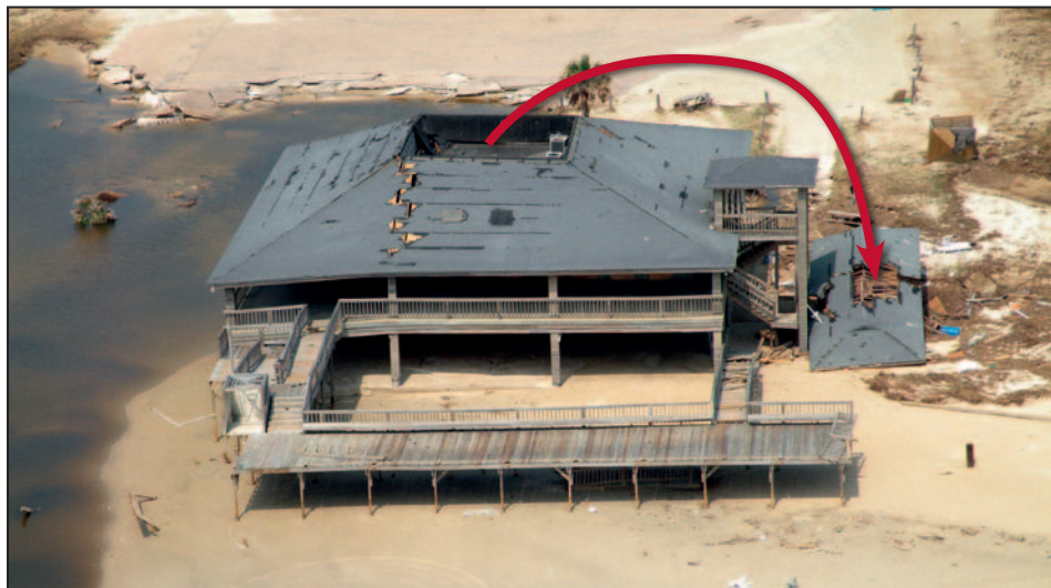
Figure 3-10. Beach house with roof structure removed by Hurricane Ike (Galveston, TX, 2008)
