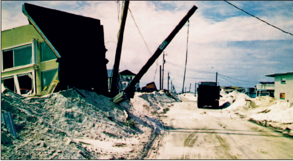
Figure 3-50. Overwash from Hurricane Opal (1995) at Pensacola Beach, FL, moved sand landward from the beach and buried the road, adjacent lots, and some at-grade buildings to a depth of 3 to 4 feet
