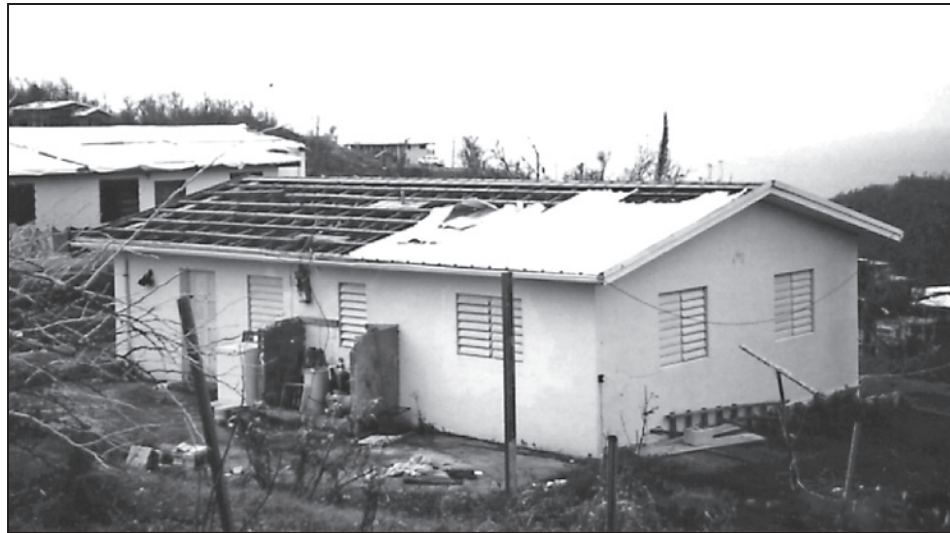
Figure 2-6. This house lost most of its metal roof covering due to high winds during Hurricane Marilyn in 1995 (location unknown)
