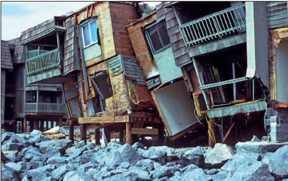
Figure 4-23. Damage to buildings sited behind a rock revetment close to an eroding shoreline at Garden City Beach, SC (Hurricane Hugo, 1989)
