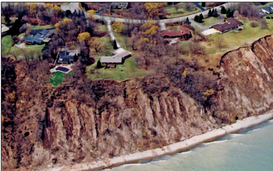
Figure 3-46. Long-term erosion of the bluff along the Lake Michigan shoreline in Ozaukee County, WI, increases the threat to residential buildings outside the floodplain (1996 photograph)
