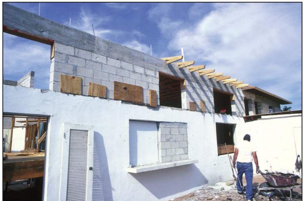
Figure 67 The extended first-story walls.
