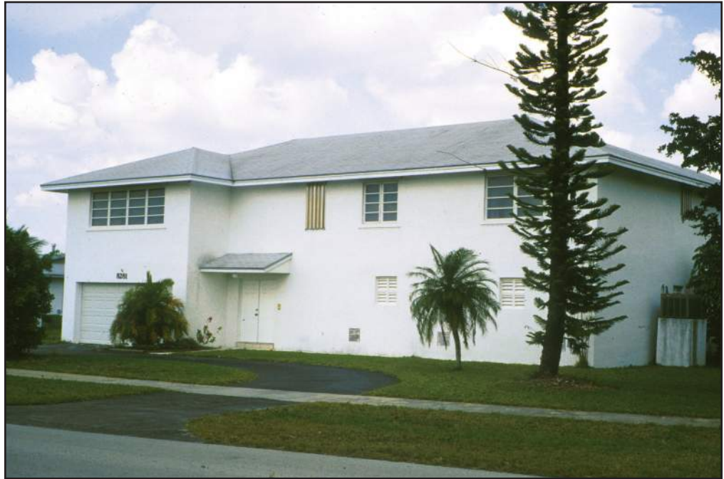
Figure 64 From the outside, the completed house, with its stucco walls, looks like a conventional masonry house.
