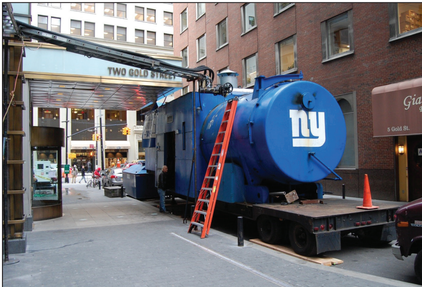
Figure 3-7. Portable boiler provides heat during repair of flood damage.
