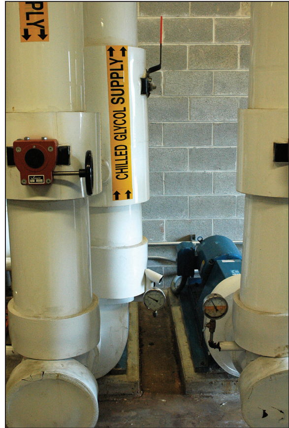
Figure 5-4. Chilled water pump, Georgetown, Delaware.
